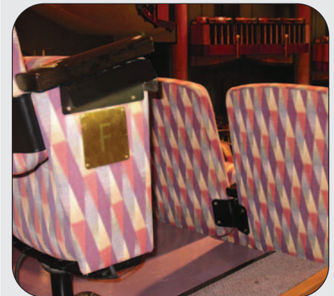
Tivoli lights are placed under seat armrests to help illuminate row letters.
