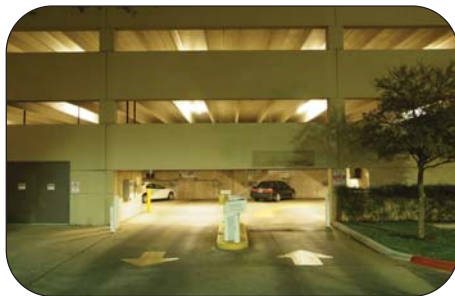
Entrance to Parking Structure in Austin, TX with BetaLED Luminaires
