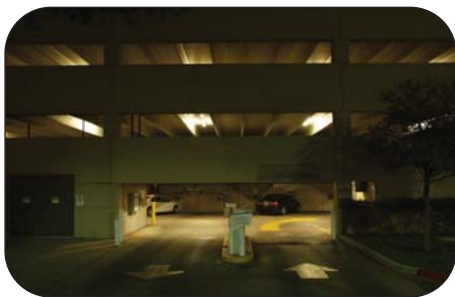
Entrance to Parking Structure with Traditional Fluorescent Strip Lighting
